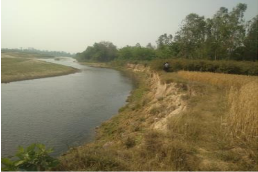
Figure 7: Bank erosion and cereal crops along Patharaiya banks at Joshipur-4, Dahabariya
