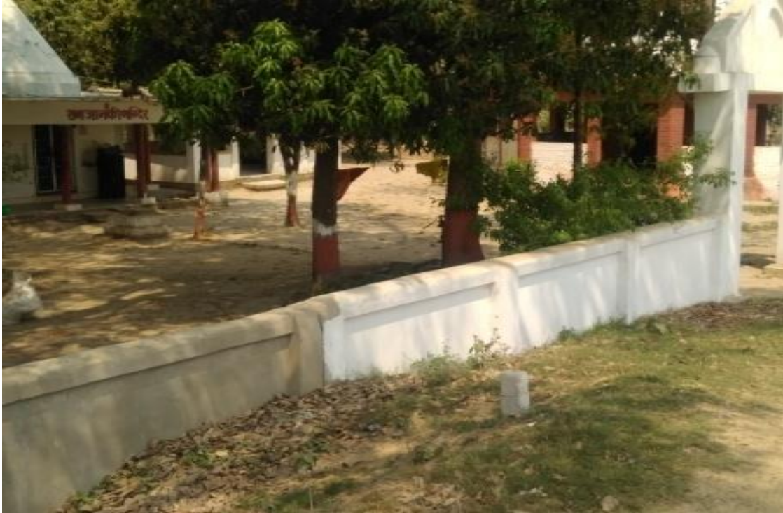
Concrete pillar demarking embankment area near Shiva Mandhir at Joshipur-4, Bani
