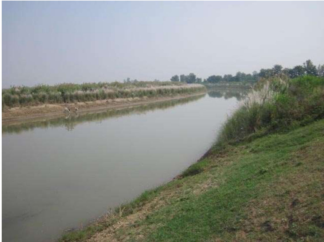
Naya Basti Baidi embankment with rich vegetation on embankment
