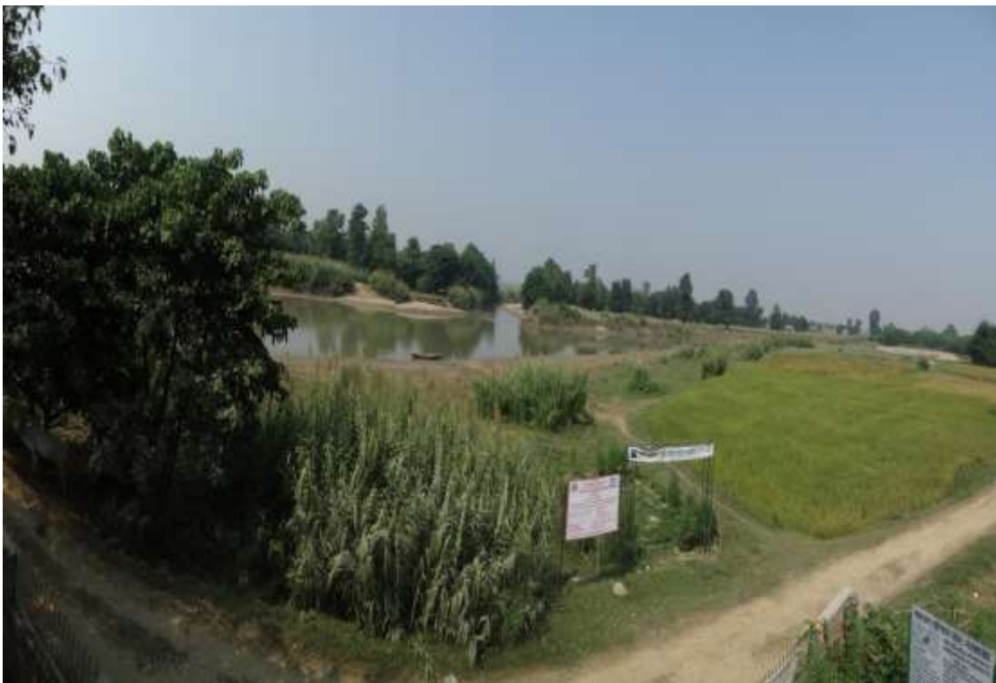
Dhungana Tole, the confluence site of Kanda and Pathraiya rivers. River embankment with civil structure.
